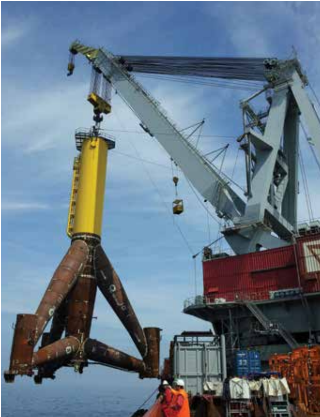
'Stanislav Yudin' installing a tripod for Borkum West II
