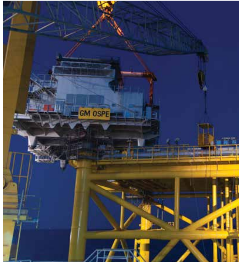
'Oleg Strashnov' installing a substation for Gwynt y Môr
