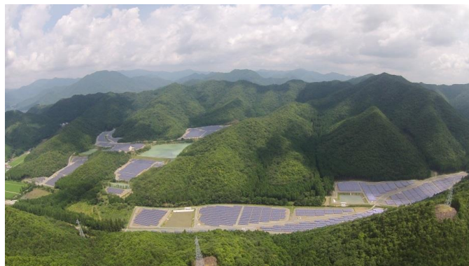
14.5MW solar power plant in Taka Town, Hyogo Prefecture of Japan
