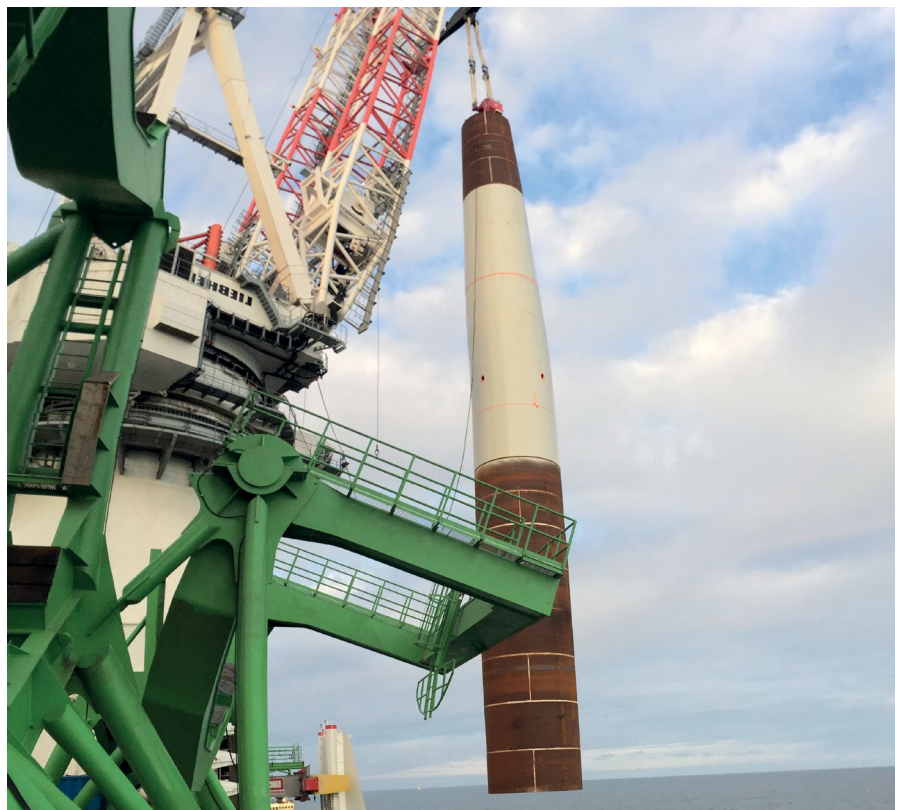
A Monopile installation
