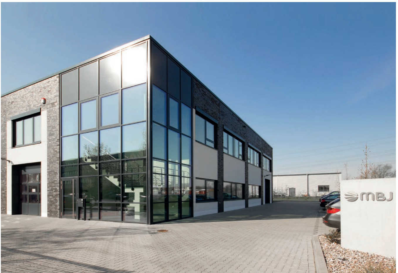
Figure 8: MJB Solutions GmbH headquarters
