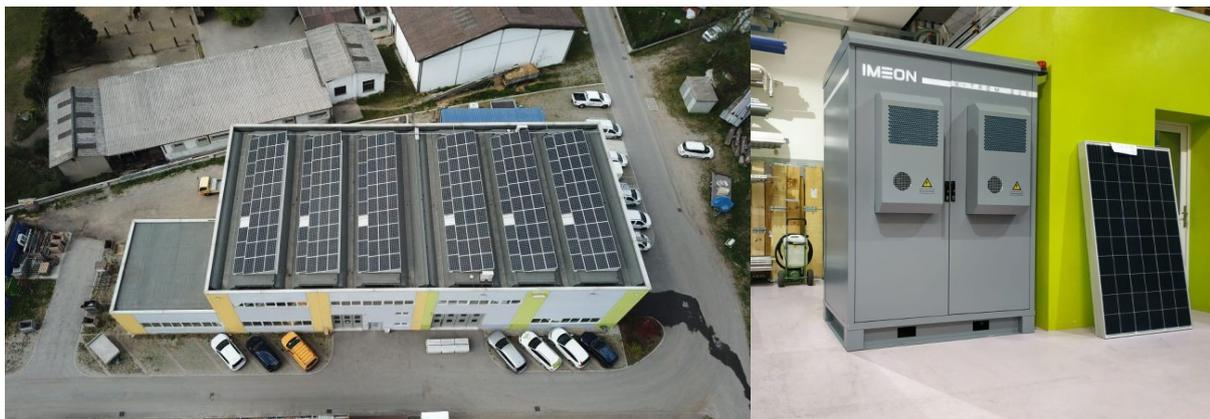
In December 2014 the company invested in a rooftop photovoltaic installation dedicated to self-consumption. Over the years, 20% of the production of the solar installation was consumed on site and 80% was injected into the public grid.
